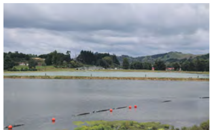
SLUDGE PONDS - TE KUITI WASTEWATER TREATMENT PLANT
