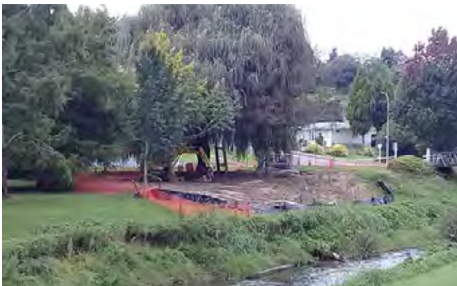
PIPE REPLACEMENT FORMING PART OF THE TAUPIRI STREET SEWER MAIN PROJECT
